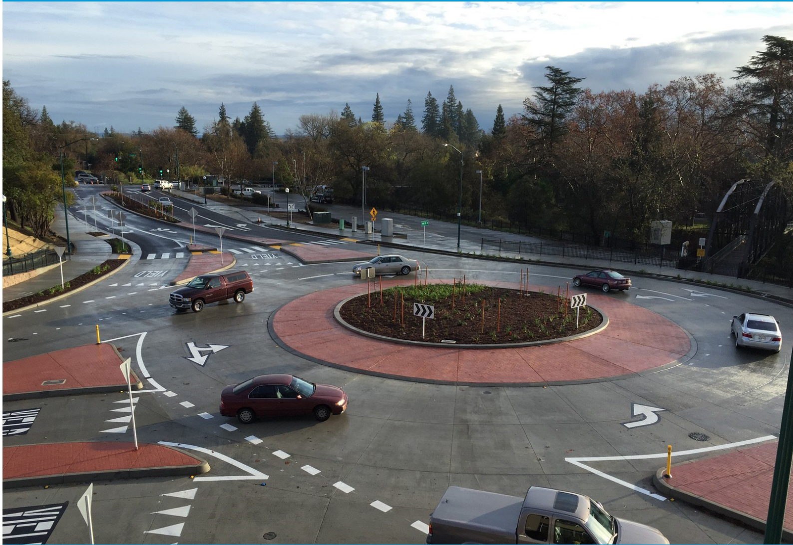
Downtown Roundabout, Roseville, California
