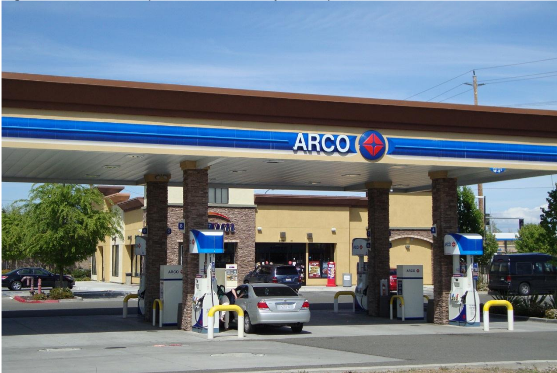
Figure 6: Arco Station (Foothills Bl. & Vineyard Rd.)
