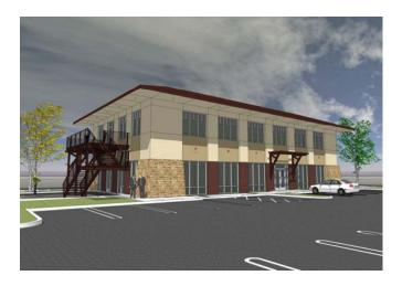
One noticeable difference between the existing and proposed buildings is that the spandrel panels on the north and east elevations have been recessed by 6 inches. At staff's request, the applicant also incorporated an additional color (Lyndhurst Timber) to be used on the recessed panels. These modifications provide additional visual interest as well as shadow and depth to the elevations.
